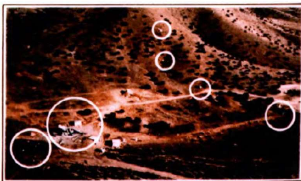
(b) Aerial View of Site after Rupture
